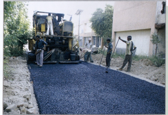
Renovation of a road
